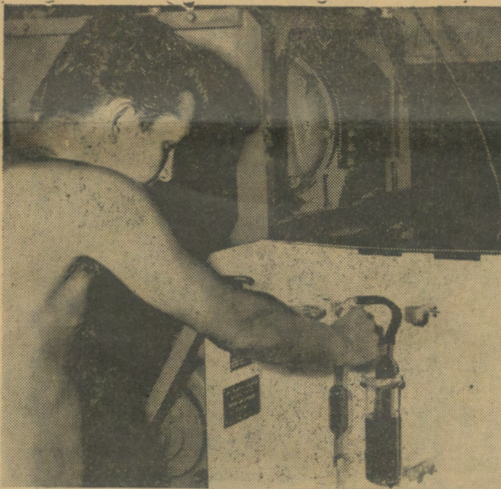
OXYGEN TEST— A2C William E. Wilson checks a sample of the liquid oxygen output for purity. Constant checks must be maintained on the material to insure it is pure and free from foreign matter, particularly hydrocarbons, which cause a violent explosion when mixed with the volatile gas.
