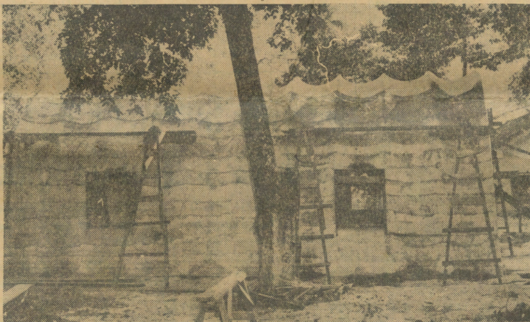
NEW HUT — The first of many huts predicted to be built in Thu Duc area. The Ctesiphon Hut is built completely of concrete and burlap, supplied by USOM. The building is being done by the Popular Forces soldiers guided by American advisors.
