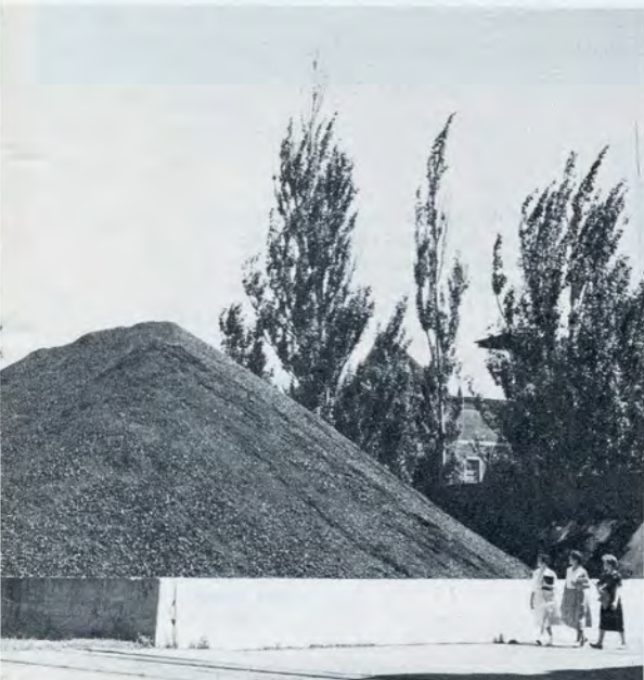
Piled nearly as high as the trees is this 10,000 ton supply of coal. The stockpile, located near the power plant, will last 30 days in the middle of winter.
